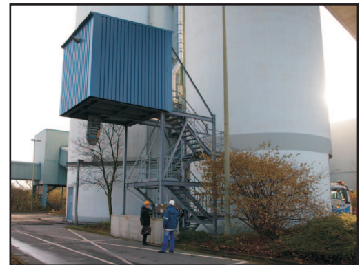
New Truck Loading Station
